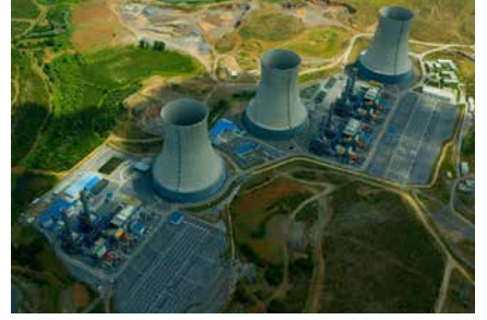
Enka Power Plant – Erbil – Süleymaniye
