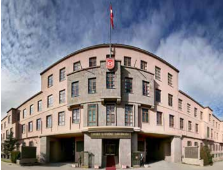
MINISTRY OF NATIONAL DEFENSE COMPUTER CENTER SERVER ROOMS - ANKARA
